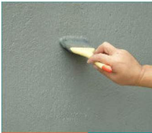
WATERPROOFING 2K COATING
