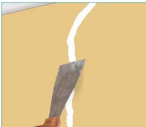
CRACK FILLING
